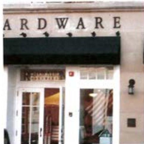
Fixtures with historical character illuminate the first floor walls and adjacent sidewalk.
