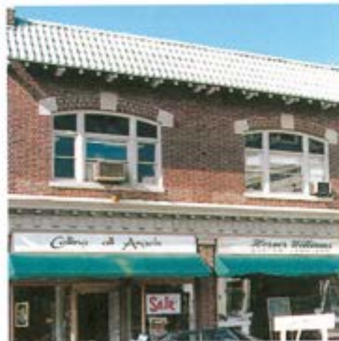
Wide flat arches in upper floor windows can be appropriate above a simple shop front design.
