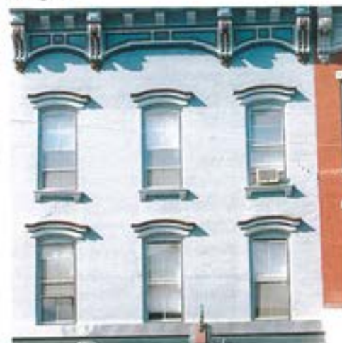
Some punched windows can include very flat arches but not round ones.
