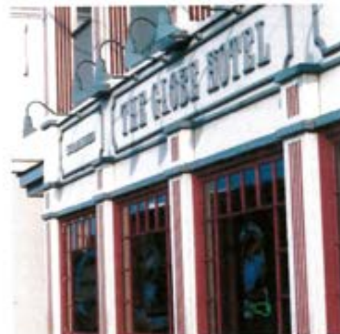
Painted fixtures enhance lights as part of façade both day and night
