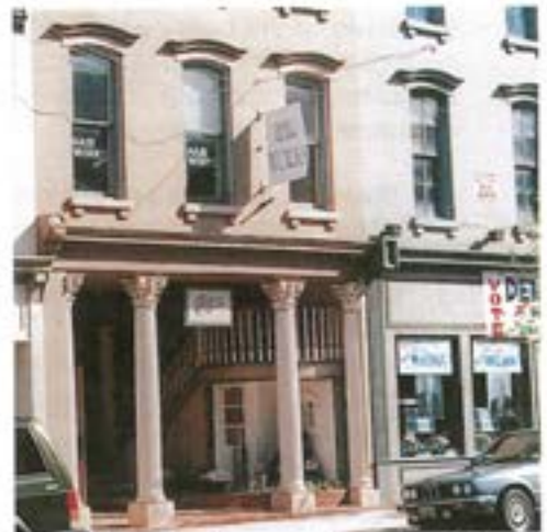
Painted wood columns and cornice with painted brick
