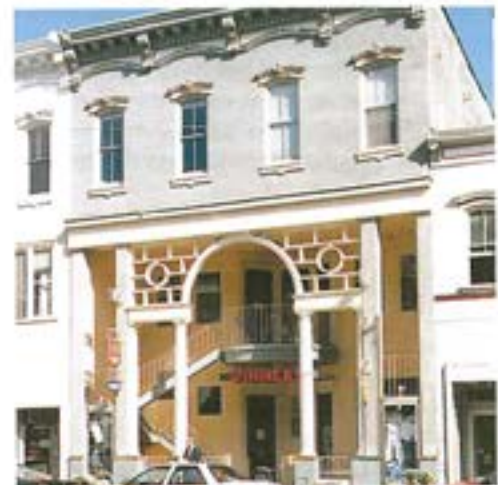
The front façade is at the sidewalk, but the inner façade is set back
