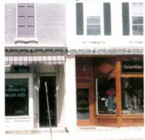
Two shop fronts that are well-proportioned and compliment the facades above
