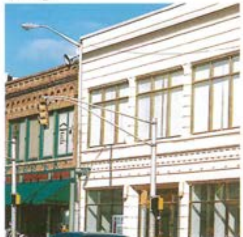
Windows filling the spaces in the building frame
